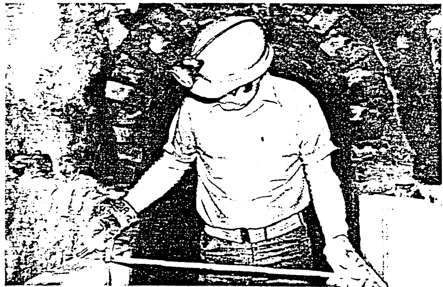
A St. Paul City Sewer Maintenance worker makes repairs on an old portion of storm sewer in downtown St. Paul.
