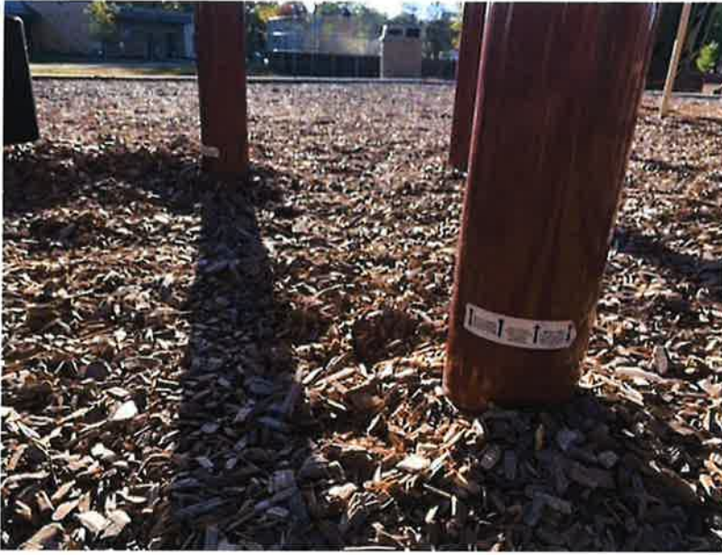
These wood chips are too low; they are supposed to be up to the white tag.
