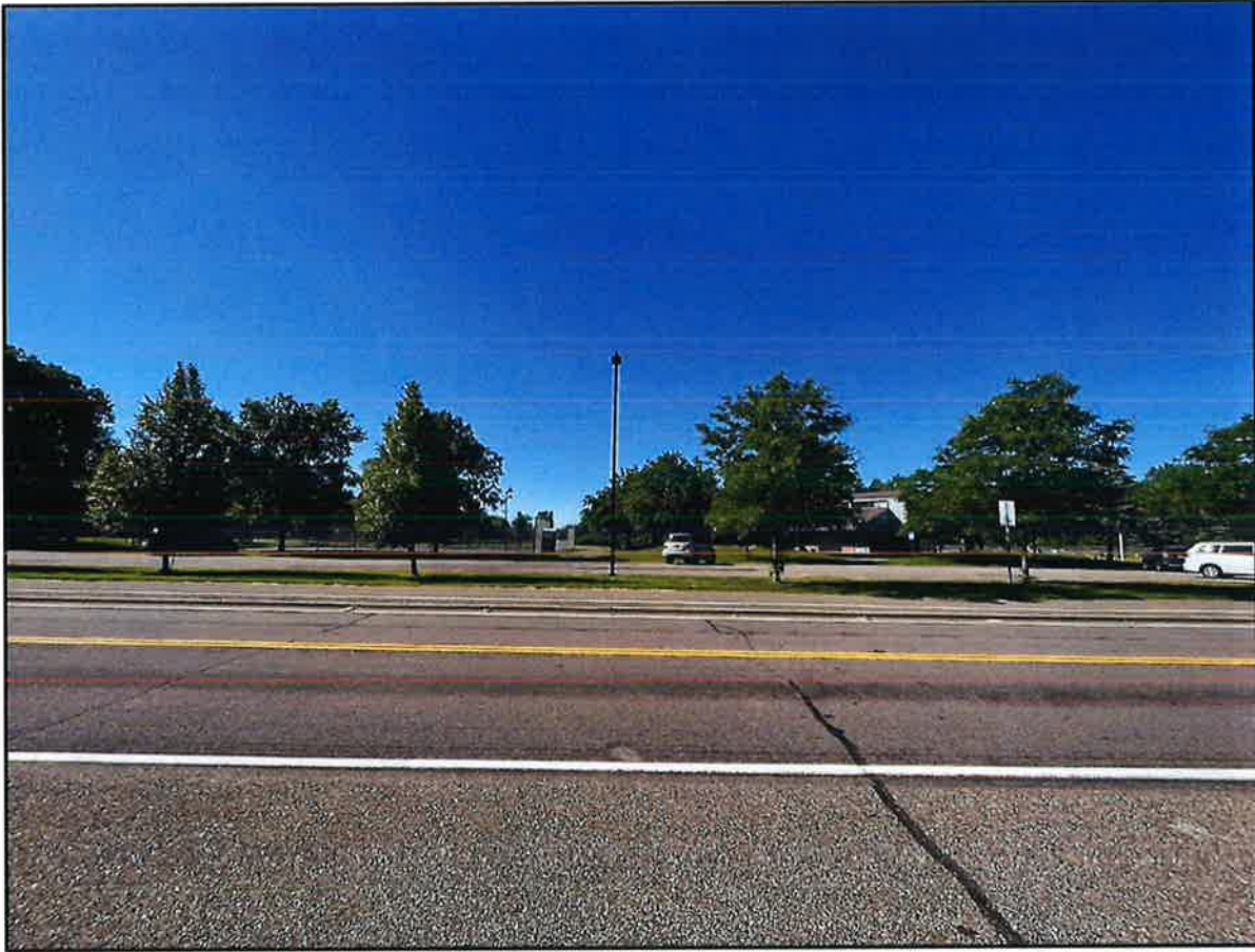
SOUTH VIEW OF SUBJECT PROPERTY AS SEEN FROM ROSELAWN AVENUE WEST
