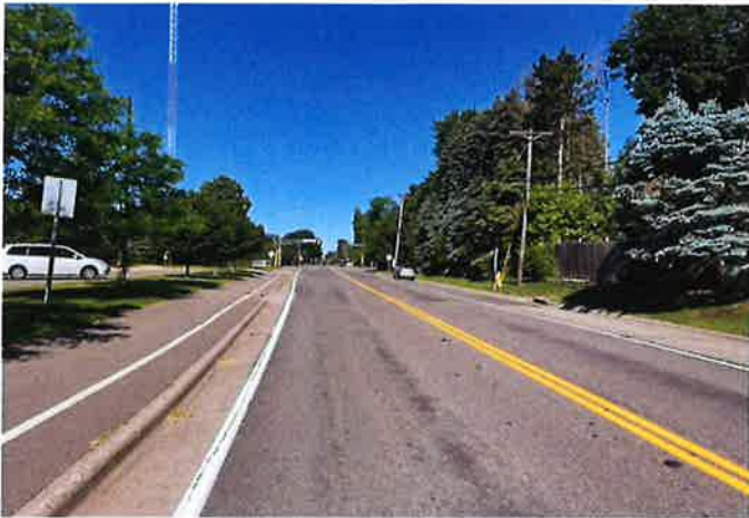
West view of Roselawn Avenue West.
