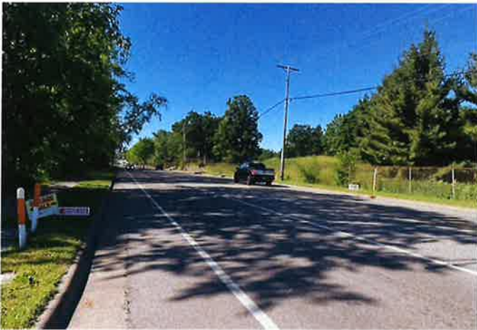
South view of Cleveland Avenue North.
