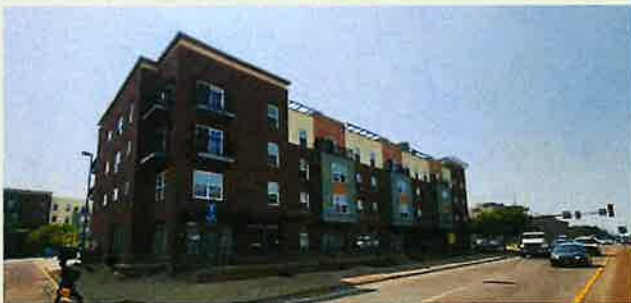
TOWN SQUARE APARTMENTS/FALCON HEIGHTS SENIOR APARTMENTS (1550 LARPENTEUR AVE W)
