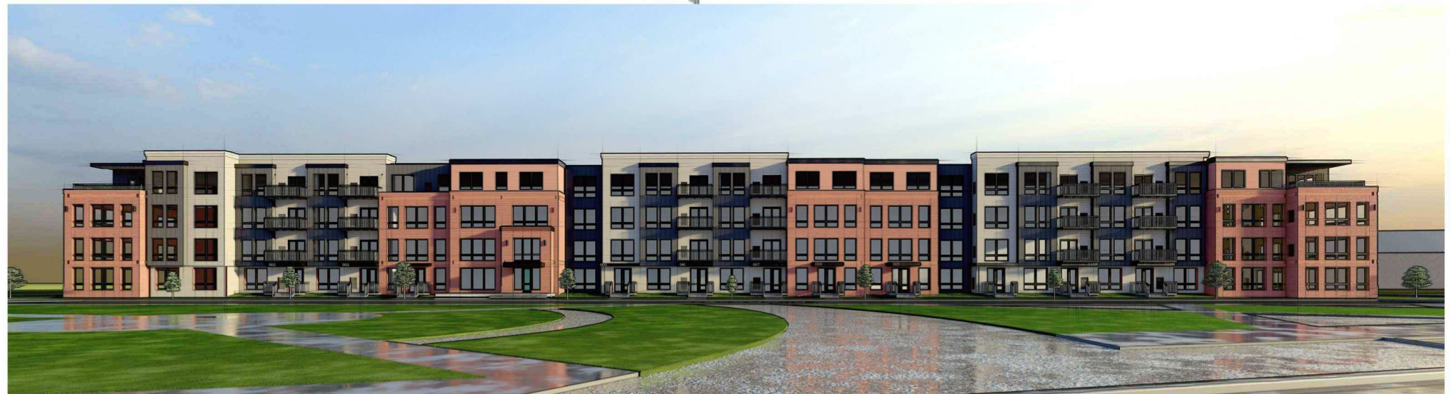
NORTH ELEVATION OF THE MULTI-FAMILY BUILDING
