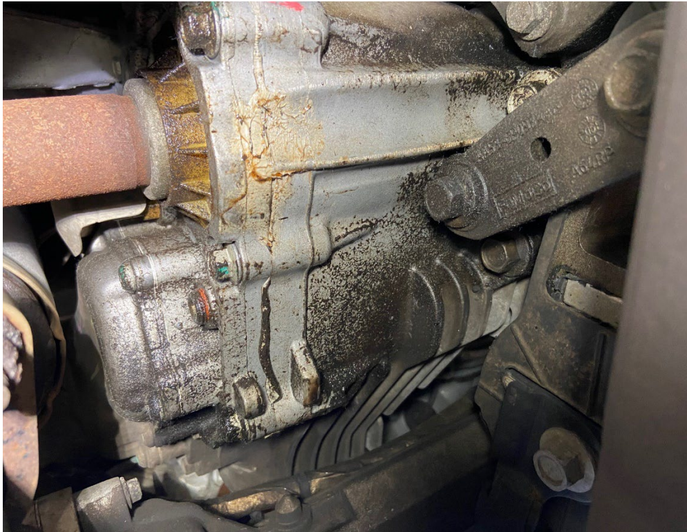
The PTU has a small leak and may need replaced at some point in the future.
