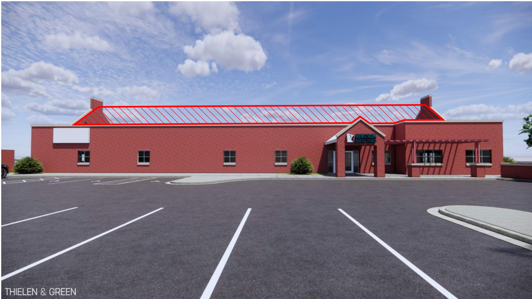
OPTION 1 - KEEP EXISTING PARAPET (PROVIDE STEEL BRACING BACK TO ROOF DECK)
