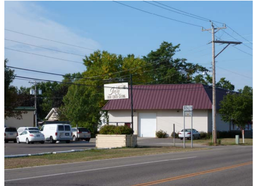
Telephone/power poles along TH-5
