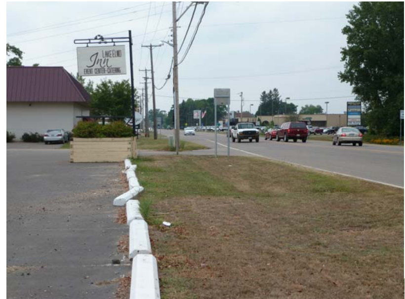
Lake Elmo Event Center ditch looking west
