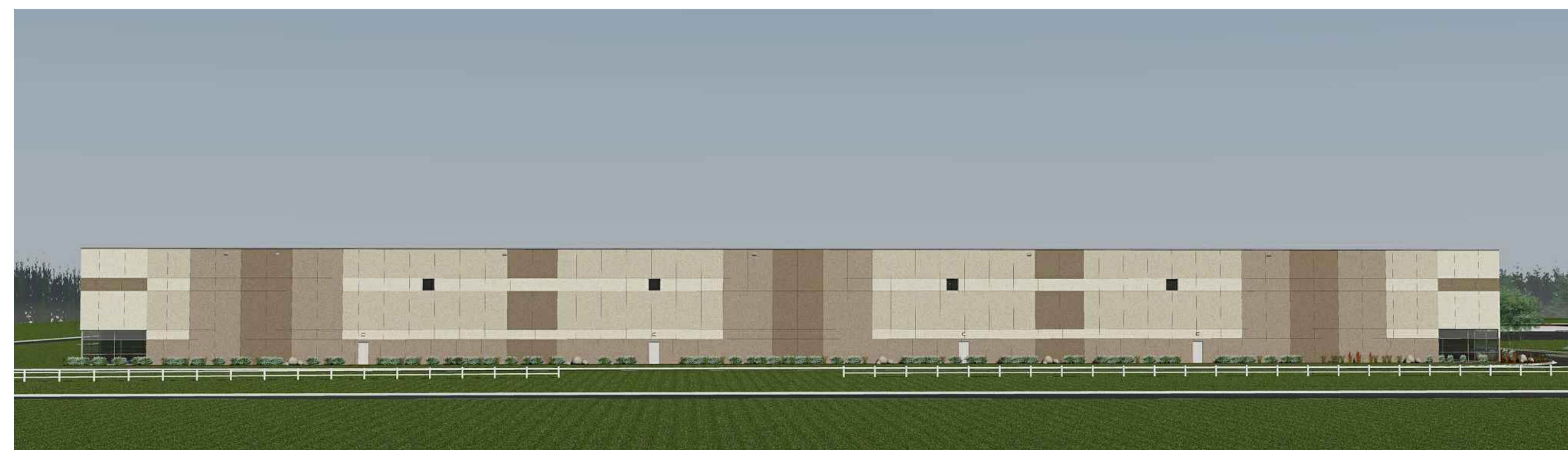
View from West - Phase I Building
