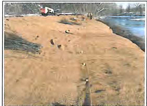
Woven 100% natural fiber erosion-control materials being utilized along a central Minnesota stream. ©MN DNR, Nick Proulx
