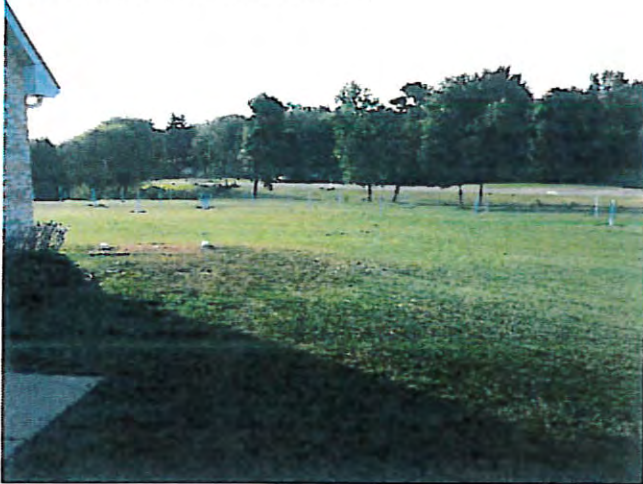
Septic Drain Field from Driveway
