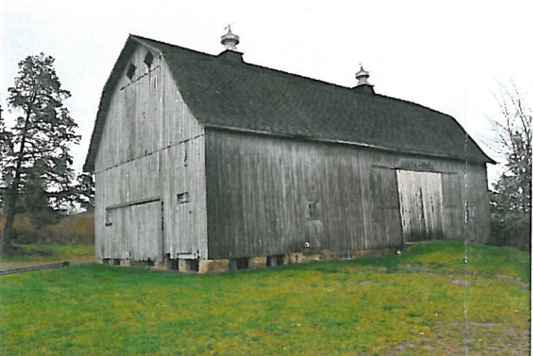
EXISTING BARN VIEWED FROM NORTHWEST
