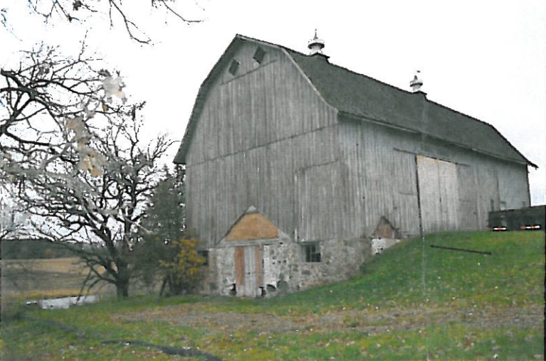
EXISTING BARN VIEWED FROM SOUTHEAST
