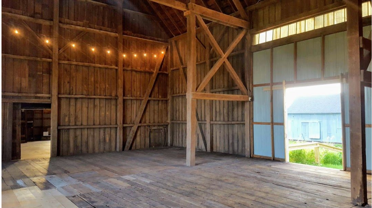
The inside of the historic barn is clean, open and beautiful, with old timber and mortise and tenon construction. The plan is to keep this available to tour, and most likely to set up a history display relating to the farm, but not use this regularly as a meeting space.
