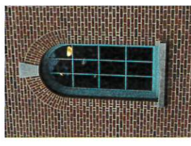
PAINTED METAL CLAD WOOD WINDOWS, WITH SILLS AND BRICK ARCHES
