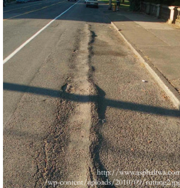
Rutting, Distortion
