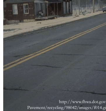
Transverse Cracks
