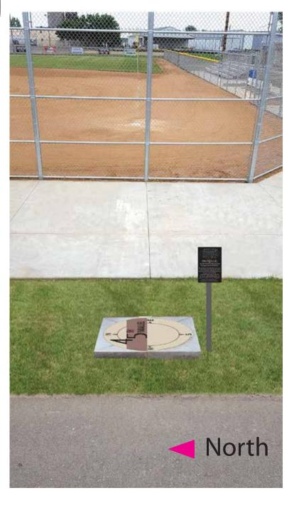
27" in Diameter disc - cast specialty concrete - flush mounted into a concrete pad constructed in the grass strip between the walking path and concrete gallery.
