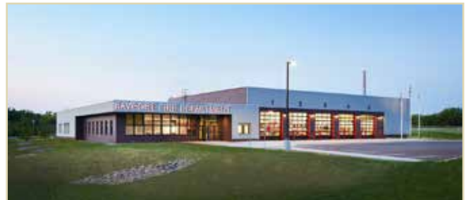
BAYPORT FIRE STATION Bayport, MN
