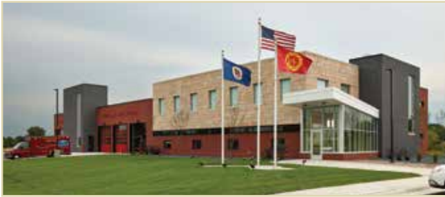
CENTRAL FIRE STATION Cottage Grove, MN
