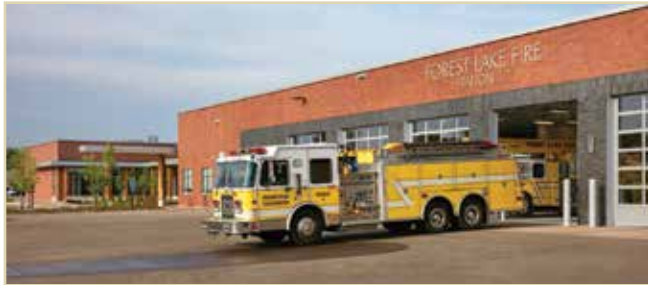
FOREST LAKE PUBLIC SAFETY BUILDING AND CITY HALL Forest Lake, MN
