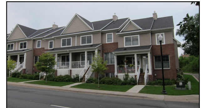
Attached units on a public street benefit from individual entries.
