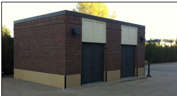
Trash and utility areas should be located out of the view of the right-of-way and screened using materials that match the principal structure.
