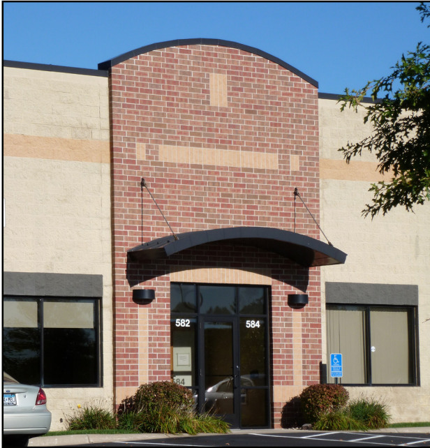
Canopies and changes in building materials help accentuate entryways.
