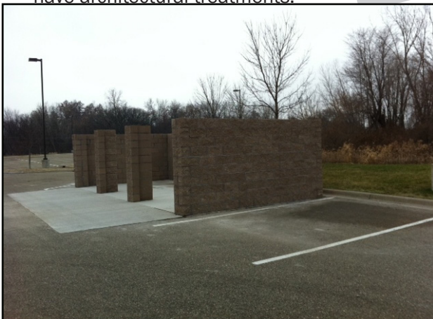
Garbage collection areas should be located to the rear of the site and screened using materials that match the principal structure.
