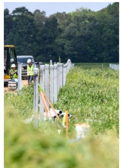
Figure 3. Steel pile installation
