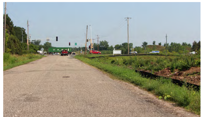
Existing Manning and MN 36 intersection.
