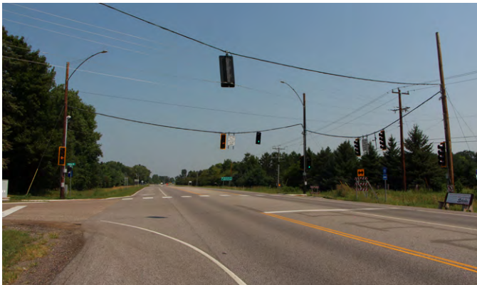
Signalized intersection at County Road 15 and 50th Street.
