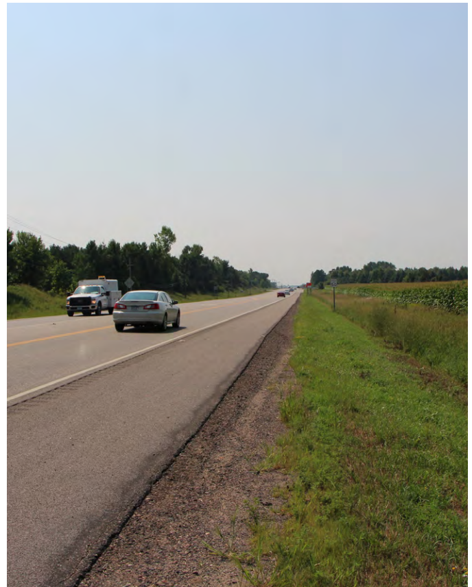
Typical road section of County Road 15 looking south.
