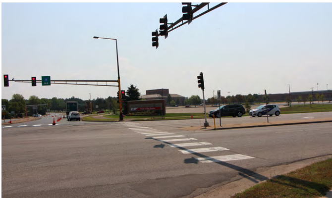
Signalized intersection at County Road 15 and 58th Street.
