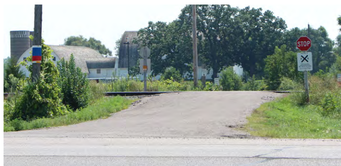
Existing at-grade railroad crossing in Lake Elmo Park Reserve.
