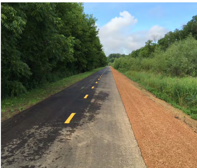
10-foot regional trail with limestone shoulder.
