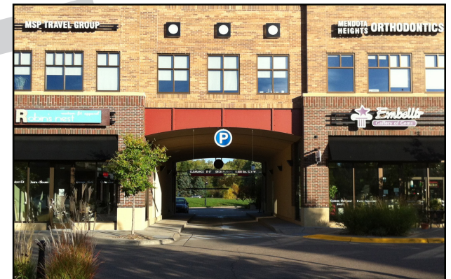
Parking is encouraged in the rear of the site to accentuate front building elevations.
