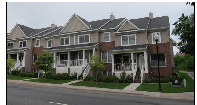
Attached units on a public street benefit from individual entries.
