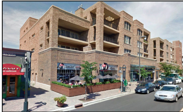
Brick is a high quality material that is consistent with an old downtown mixed-use area.
