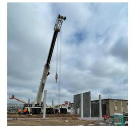
Precast concrete wall panels arrived on site this week and installation has begun. Rainy weather and lightning in the area stalled progress but crews will be back next week to continue work on the exterior walls.
