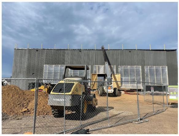
Demolition of the old roof has been completed and at least 90% of the roof has at least a temporary covering. Interior floor of the Fire Department addition is almost ready for the concrete slab to be poured. Work continues on the interior of the old building and the new main entrance.
