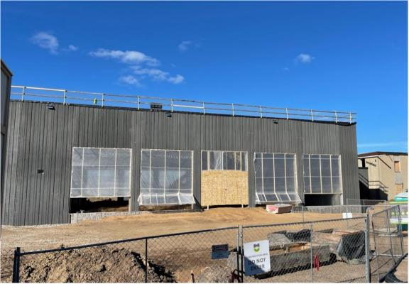
This week work focused on the roof - installing rubber membrane on the roof of the Fire Department addition and the Brookfield Building. Metal trusses were installed at the new entrance to prep that area for roofing as well.
