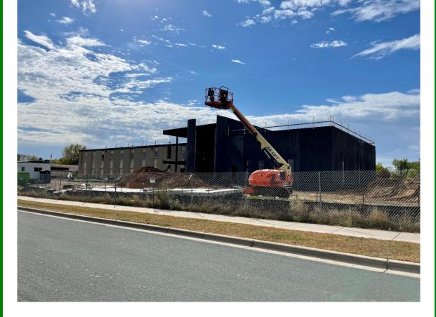
This week crews continued work on the roof areas and drain tile around the perimeter of the new additions. Work on the interior of the fire department addition will be soon.
