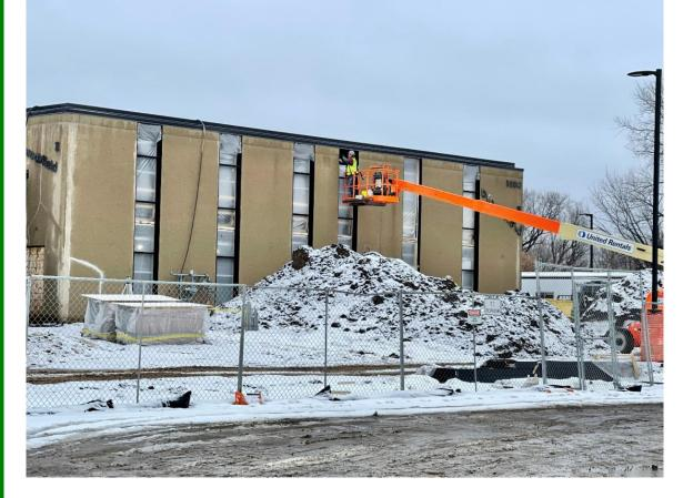
The concrete in the Fire Department apparatus bay was finished this week. Concrete was also poured for the new addition that will house the main entrance, City Council Chambers and community room. Metal window framing was installed to prep for delivery of the glass window panels next week.
