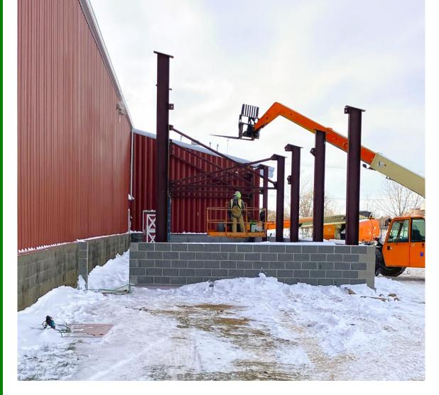
Work continued this week prepping the fire apparatus bay floor for additional concrete pours. The front of the new addition that will house the main entrance, City Council Chambers and community room is also taking shape. Out at Public Works, construction of the post frame for the building addition began this week.
