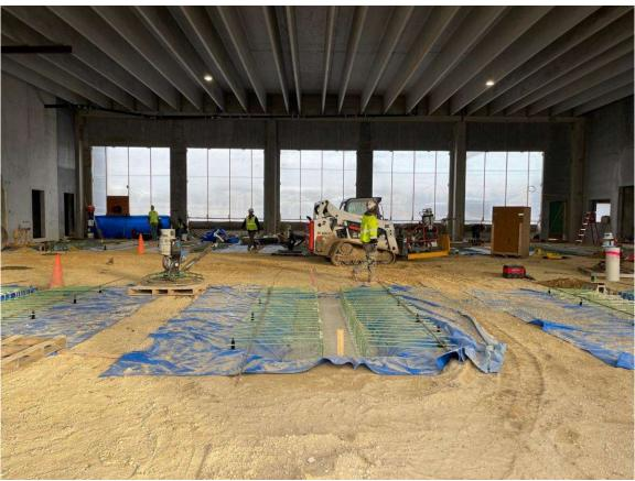
Concrete began arriving this week for the fire apparatus bay floor. Due to the size of the slab, concrete will be poured in stages over several days. The slab will be 8 inches thick when complete with highway grade concrete that is needed to support the weight of fire trucks that can weigh up to 64,000 pounds.
