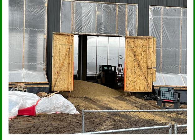
In spite of the rainy weather this week, crews made good progress this week and were busy in the fire department apparatus bays with gravel base to prepare for concrete floors to be poured. Work also continued on the northwest side of the building with installation of additional concrete wall panels.
