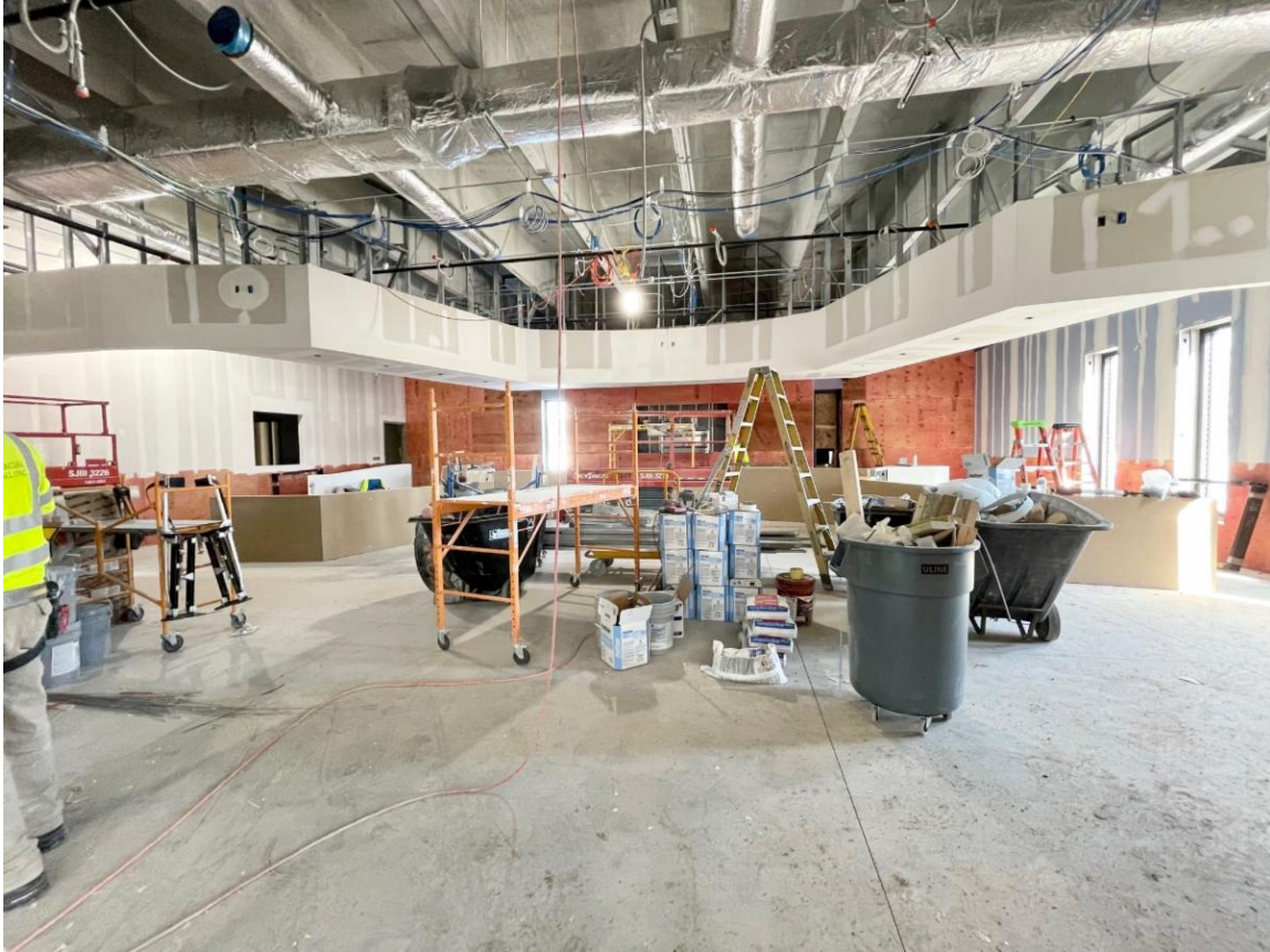
Drywall installation is in full swing in the future council chambers.
