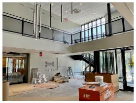
The entry atrium is looking great now that the railings have all been painted and the stairs are finished. Sound panels were installed in the Council Chambers this week and soon the City logo will be installed on the back wall. The sound panels not only look nice, but they also have sound absorbing chambers built in to help with acoustics in the room.
