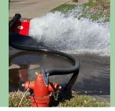
Flushing hydrants ensures the hydrants are working properly and checks for an adequate flow of water that would be needed in the event of a fire.
