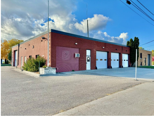
Precinct 1 - Fire Station 3510 Laverne Avenue North
