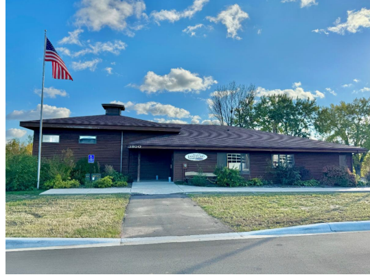
Precinct 2 - Old City Hall Building 3800 Laverne Avenue North
