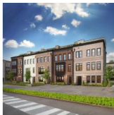
46% Classic, rear-loaded, walk-in townhouses. Half of units have turf yard and half of units have brick patios.
