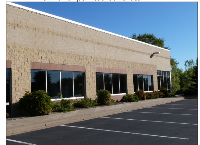
Long expanses of wall can be broken up using windows and other treatments.
