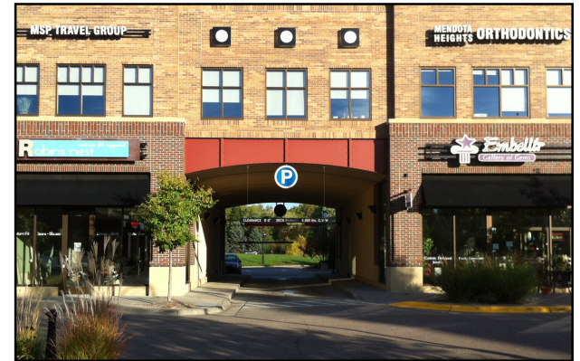
Parking is encouraged in the rear of the site to accentuate front building elevations.
