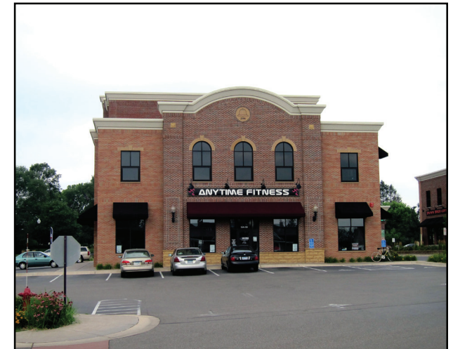
Facade articulation and windows with architectural detail add visual interest and break up long expanses of continuous façade.
