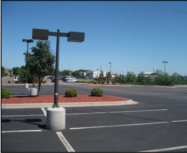
Lighting should be down-cast and shielded to prevent glare or spill-over onto adjacent properties.
