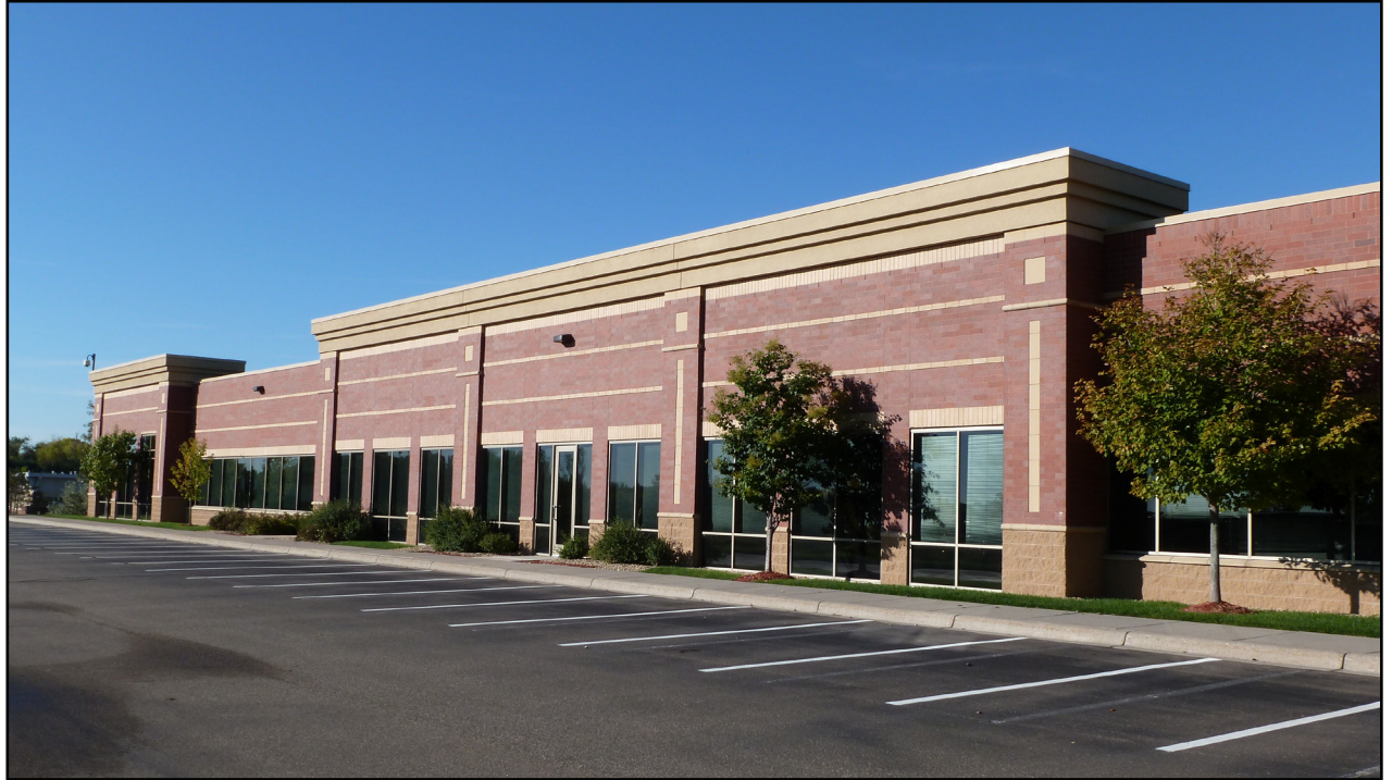
Parapets of varying height provide additional architectural detail that add aesthetic value.
