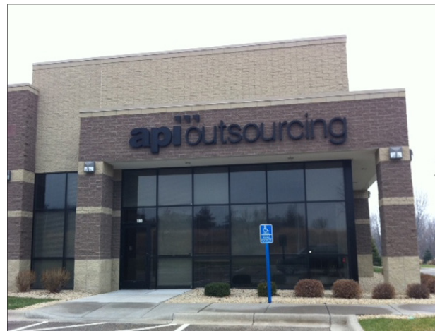
Corner treatments to larger structures add visual interest and break up monotonous design.
