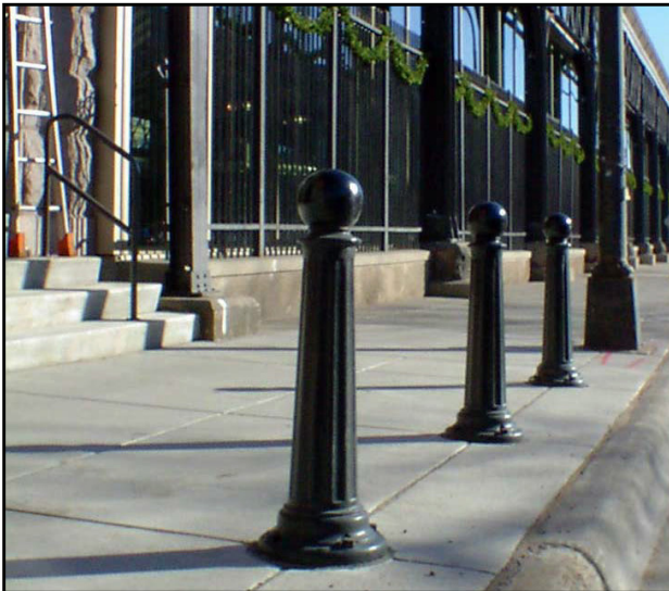
Bollards are an effective tool in delineating the pedestrian space. This style of bollard is drawn from the Lake Elmo Branding and Theming Study.
