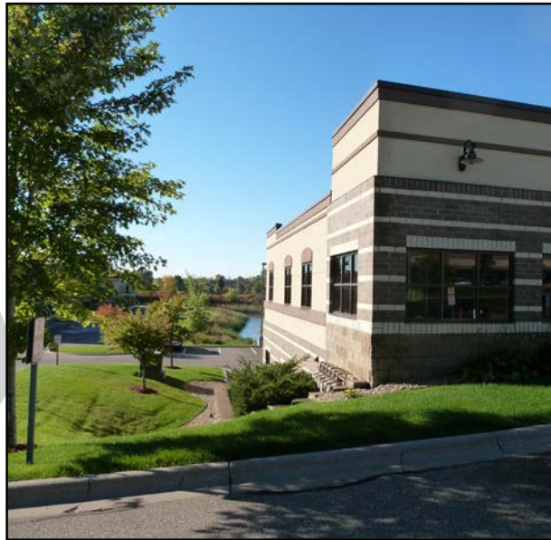
Utilizing natural topography within business park development adds aesthetic value and reinforces Lake Elmo's open space character.
