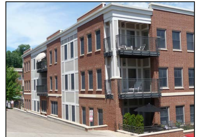
The appearance of building mass is reduced by breaking the building up into smaller sections with the use of building materials and other methods.
