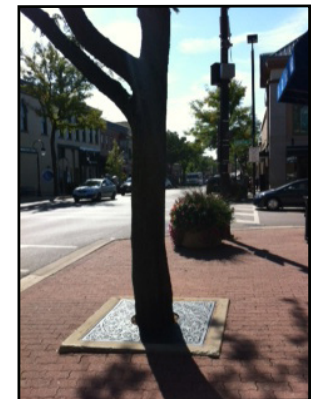
Tree gates help maximize pedestrian space in areas of high pedestrian activity.
