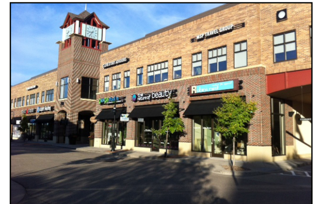
Step-down techniques and variation in building materials help reduce the scale of the building and accentuate the street/pedestrian area.
