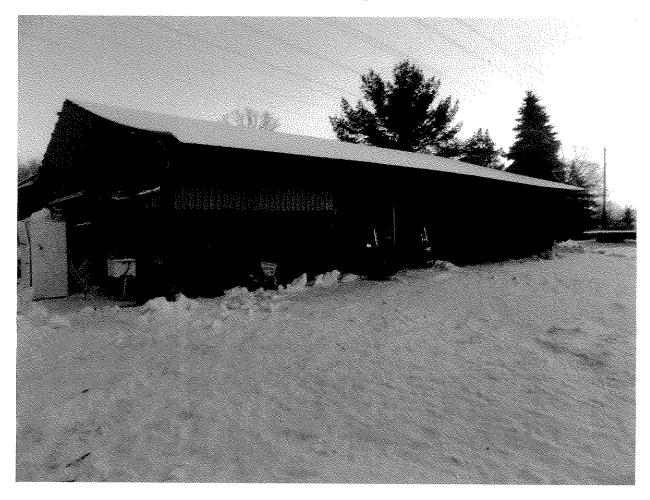
Since one third of the roof collapsed, we were told that the remaining two-thirds of the roof should be replaced and brought up to code or it could fall down too.
