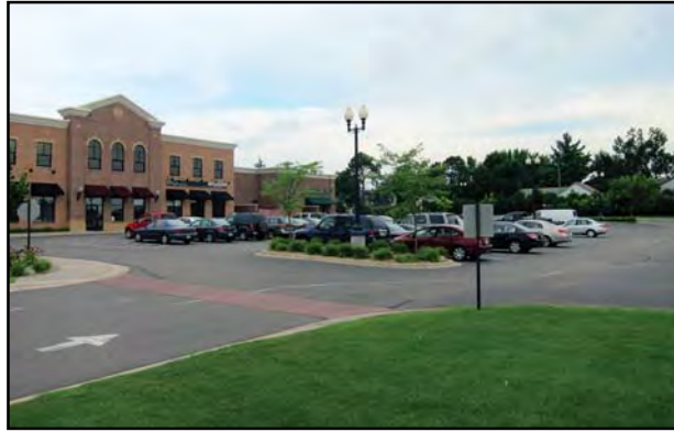
Streetscapes should include plant beds with trees to provide shade and add aesthetic value along sidewalks.
