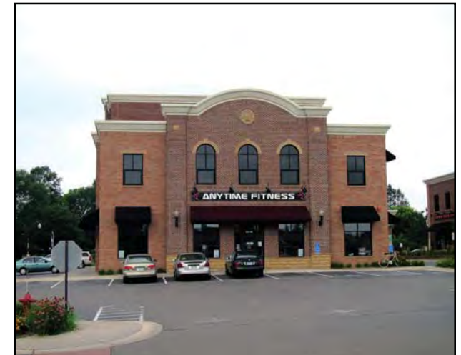
Facade articulation and windows with architectural detail add visual interest and break up long expanses of continuous façade.
