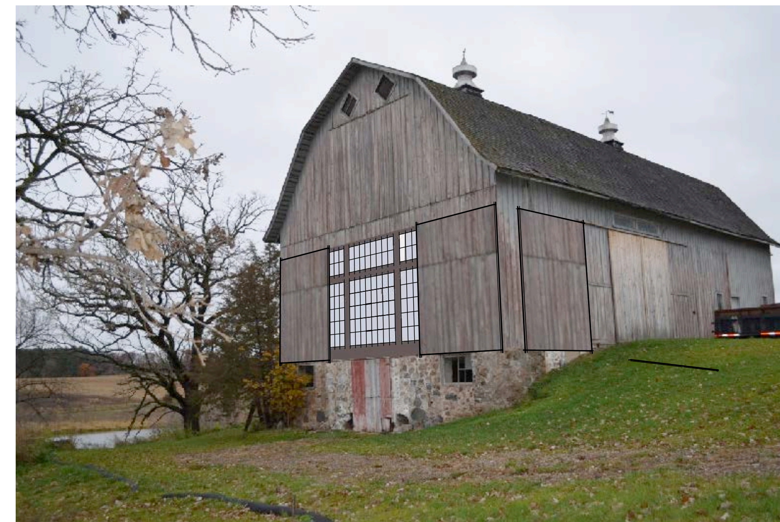
PROPOSED BARN VIEWED FROM SOUTHEAST BARN DOORS OPENED TO EXPOSE NEW WINDOWS ON SOUTH ELEVATION
