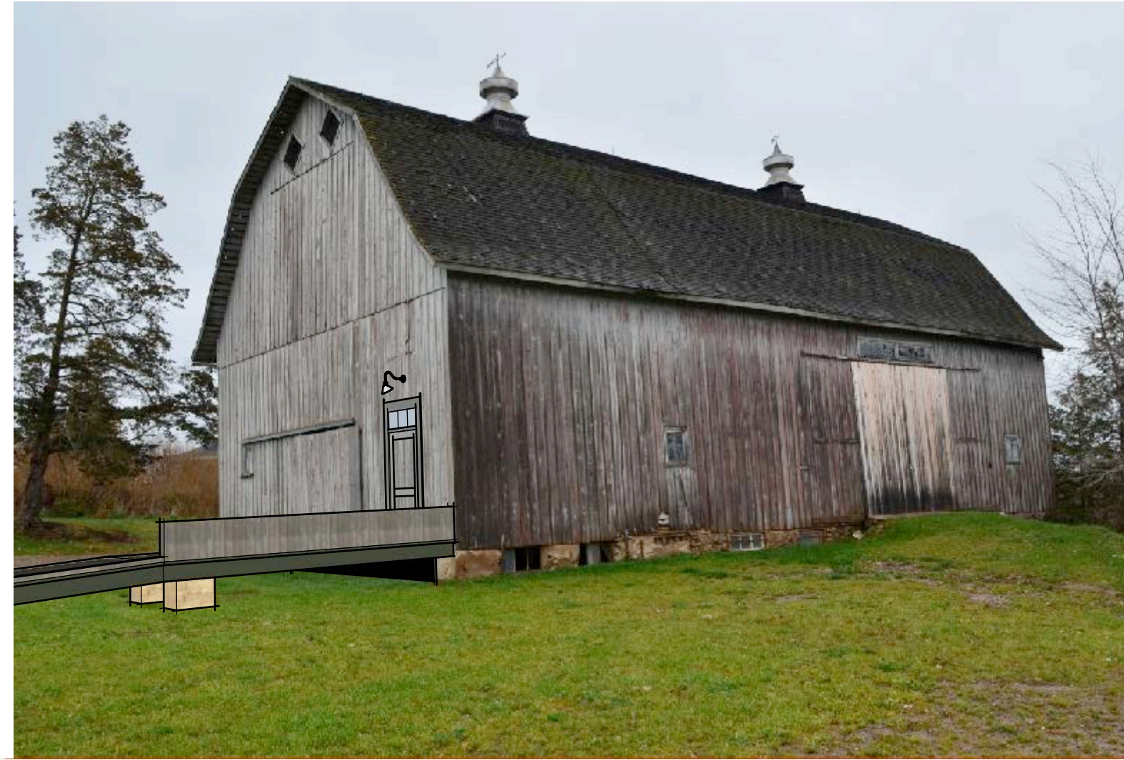
PROPOSED BARN VIEWED FROM NORTHWEST ADDED NORTH ENTRY, DECK/PATIO WITH HANDICAPPED ACCESS
