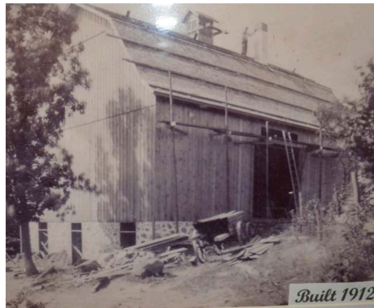
HISTORIC PHOTO OF DAIRY BARN UNDER CONSTRUCTION
