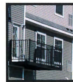
SUSPENDED DECKS & VINYL WINDOWS
