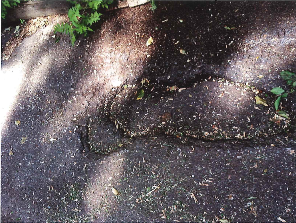
Walnut Street Alley
