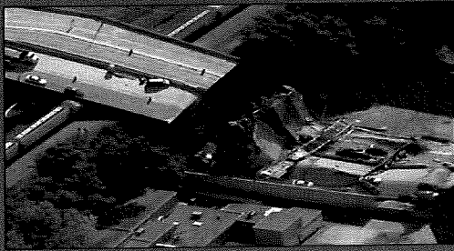
35-W Bridge Collapse 2007
