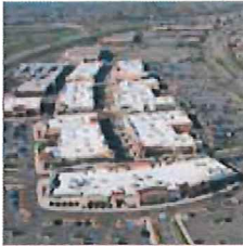
Arbor Lakes Retail Development Maple Grove, MN
