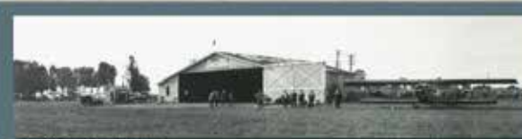
Curtiss Northwest Airport hangar
