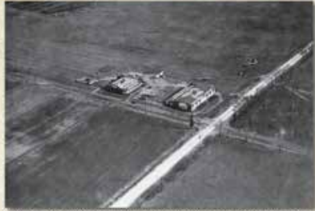
Aerial photo of Curtiss Northwest Airport and the Larpenteur - Snelling intersection. Image taken from the northwest.
