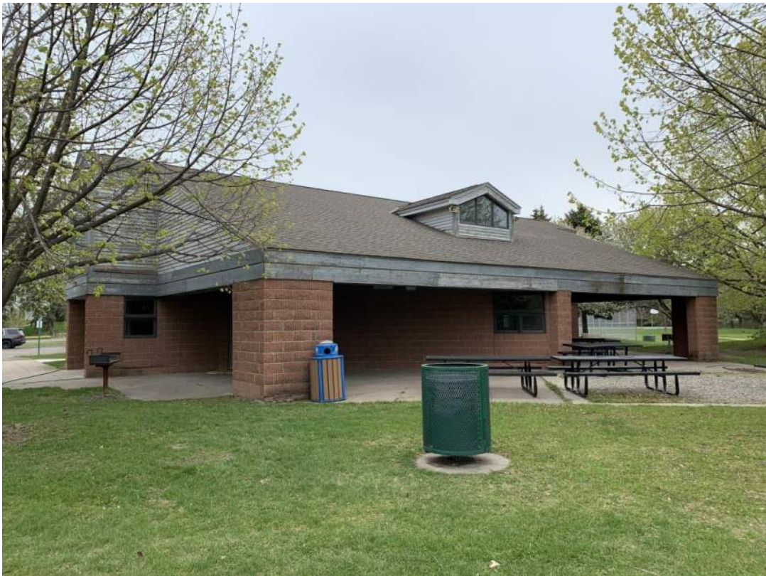
Figure 6 – Overview: Northwest Side
