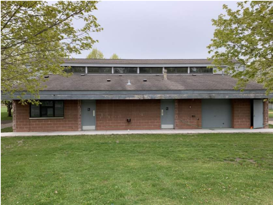
Figure 3 – Overview: Northeast Side
