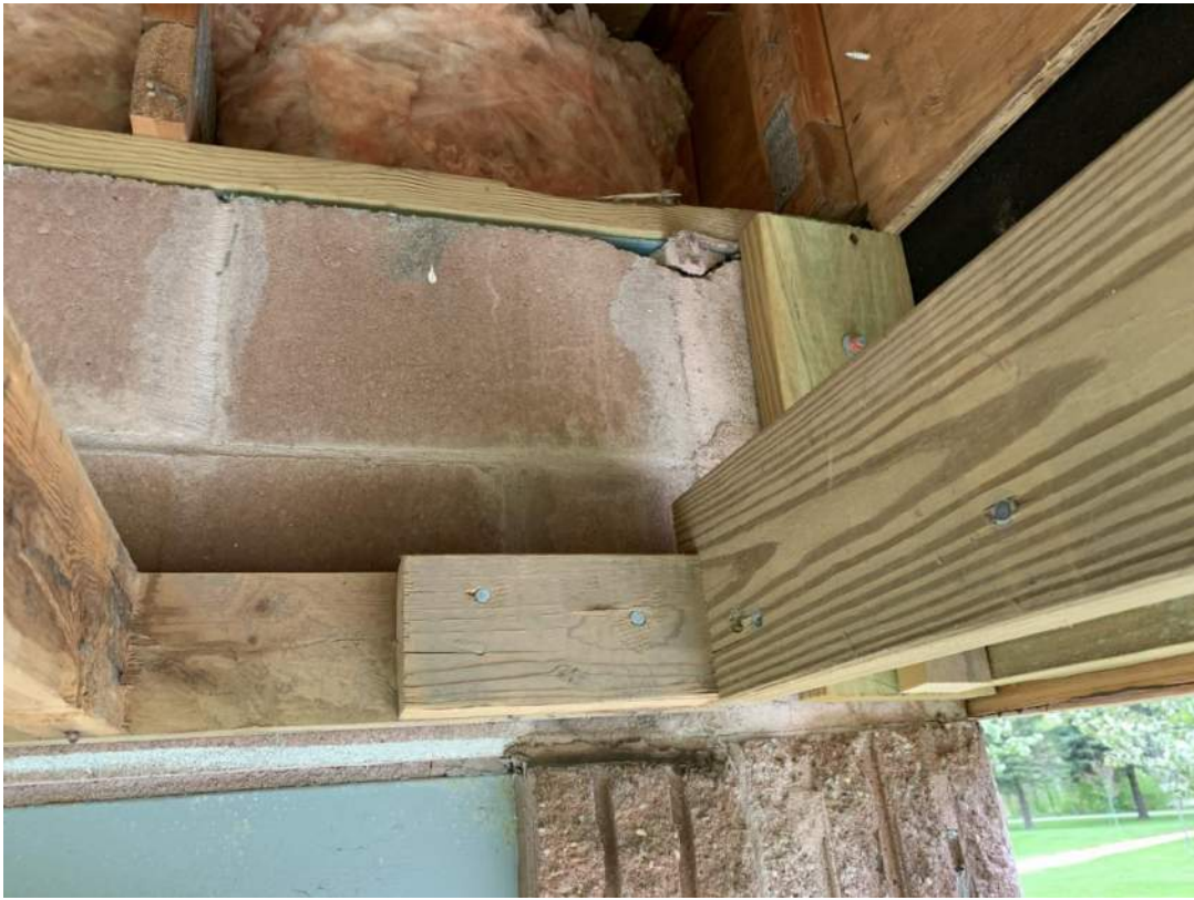
Figure 63 – S58: NE Side (Corner Breakout)
