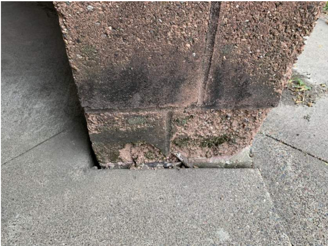
Figure 90 - N14: SW Side (Discolored Masonry)
