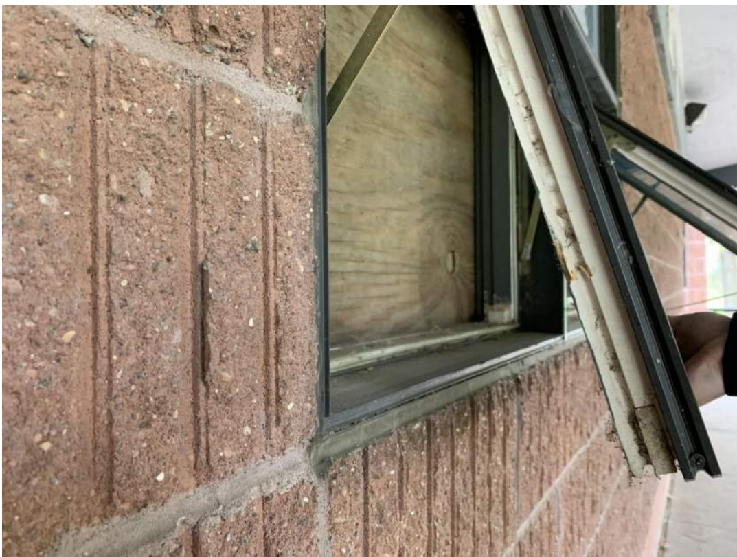
Figure 20 - S14 & S15: NW Side (Caulking)
