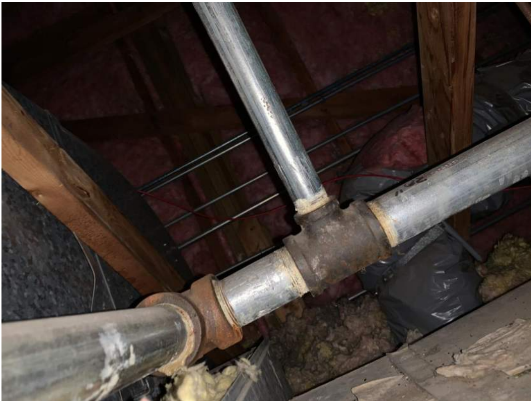
Figure 94 - N18: Interior Attic (Mouse Droppings)
