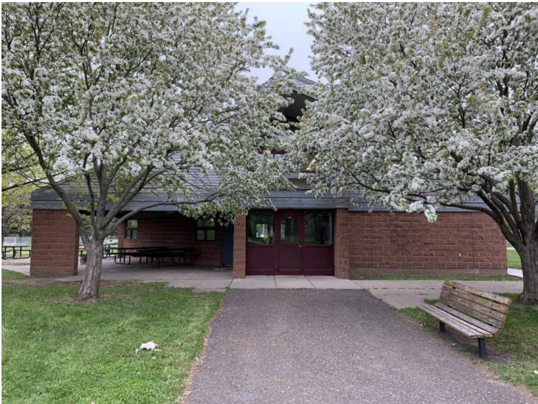
Figure 4 – Overview: Southeast Side
