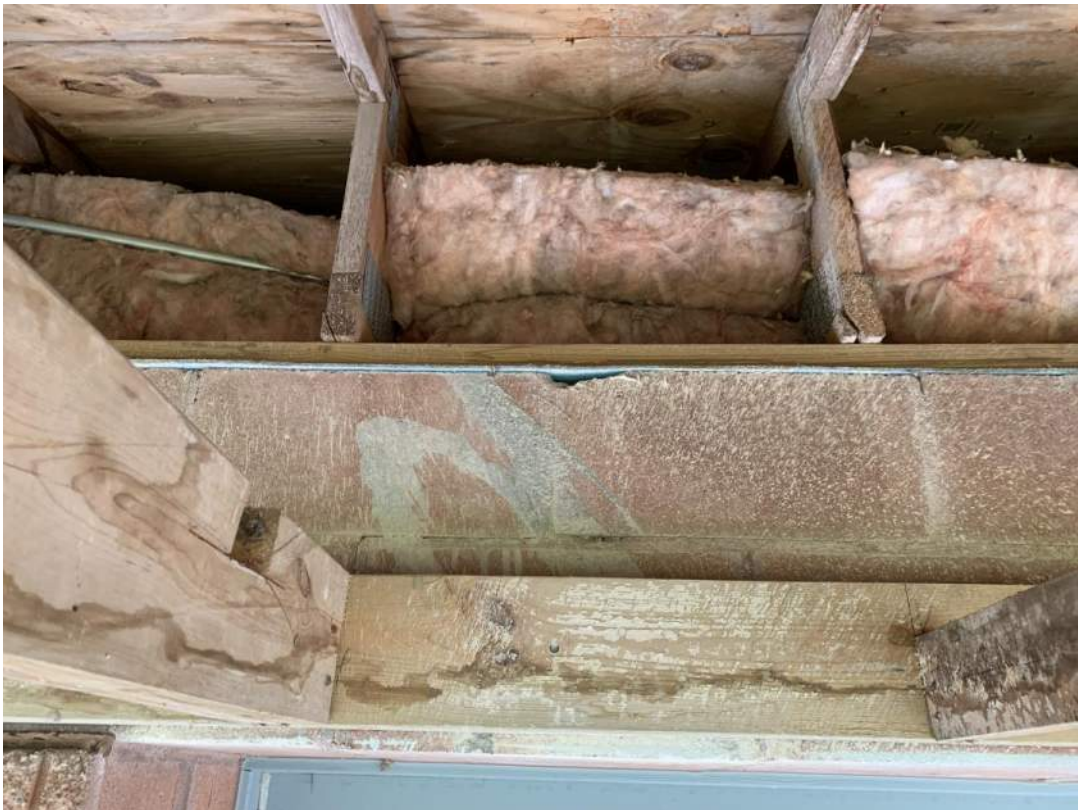
Figure 54 - S48: NE Side (Bearing Splits)
