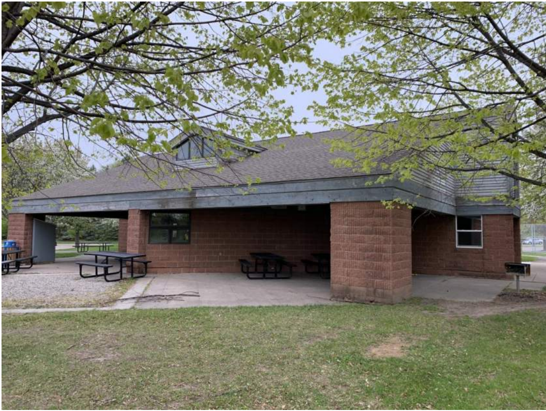
Figure 5 – Overview: Southwest Side
