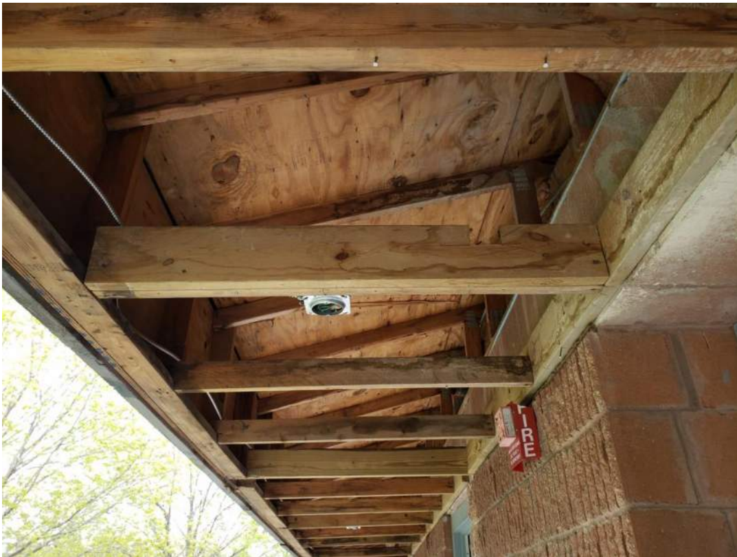
Figure 62 - S57: NE Side (Saw Cut)
