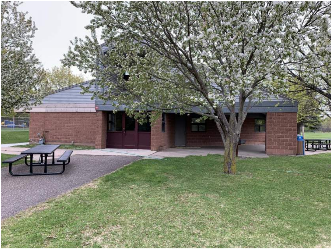
Figure 7 – Overview: Northwest Side
