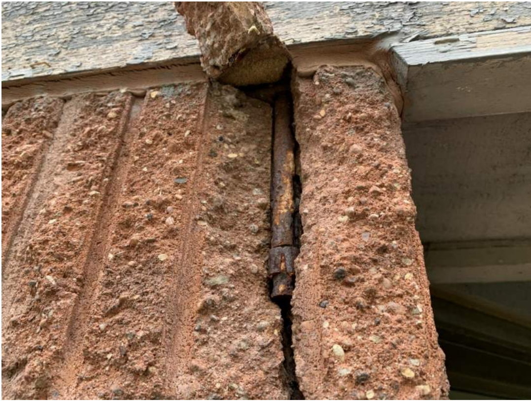
Figure 25 – S21: SW Side (Exposed Anchor)
