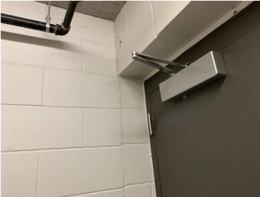
Figure 75 – S71: Restrooms (Women's Restroom Crack)
