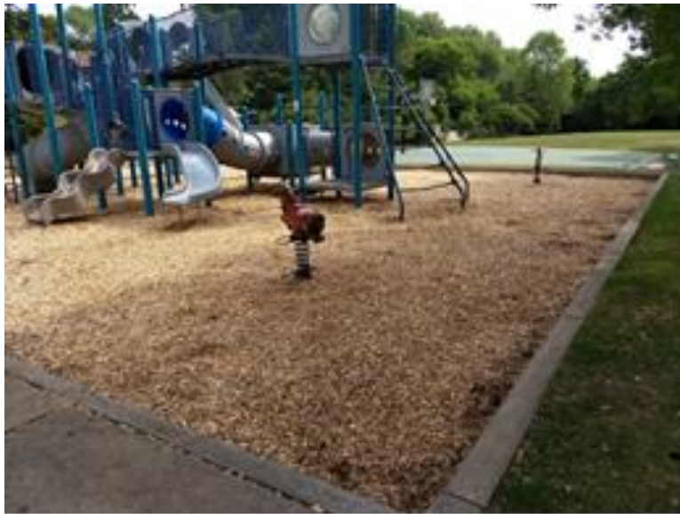
In the above photo, the wood chips are too low and the concrete curb bars access to persons with disabilities. These were common issues in all our cities.
