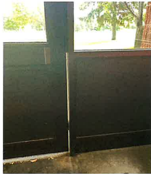
1982 original doors located at east and west entries – missing sweeps and seals
