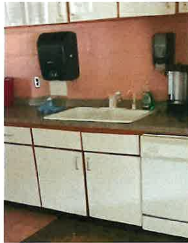
Existing Kitchen Sink
