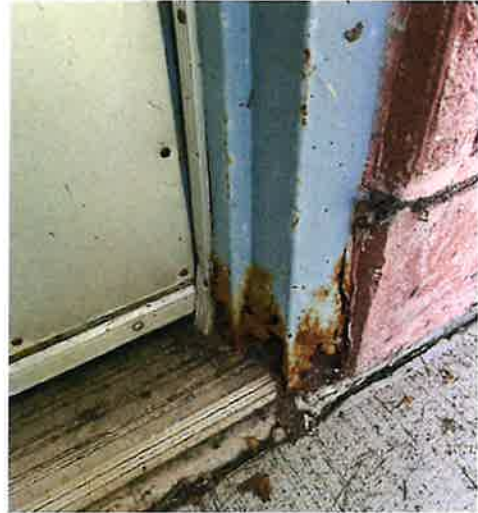
1982 original doors located on North elevation – rust damage
