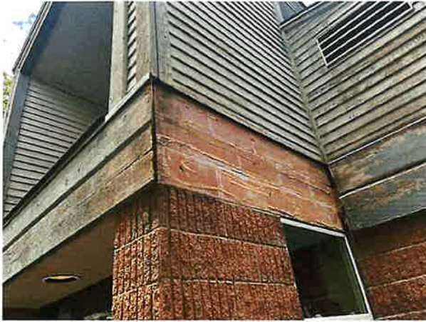
Southeast facade – Wood siding missing and paint flaking
