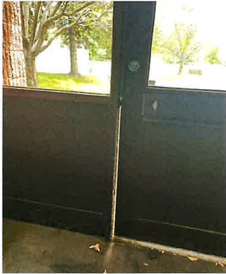
1982 original doors located at east and west entries – missing sweeps and seals
