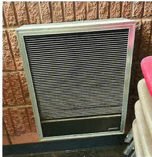
Existing in-floor duct work in main activity room and electric wall unit heaters in vestibules
